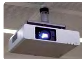
Example Ceiling Suspended Vertical Aspect (VSU) Projector Suspension Unit
